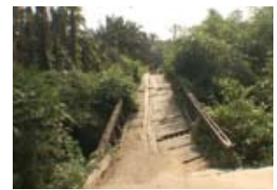
Collapsed bridge, Akwa Ibom state, Nigeria
